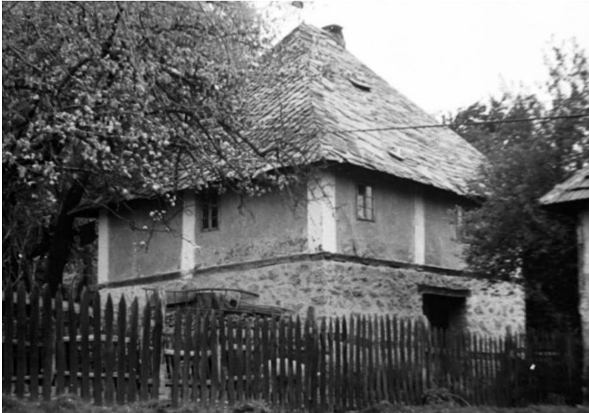
Figure 3. Adobe house on the basement, covered with stone slabs, village of Godečevo
