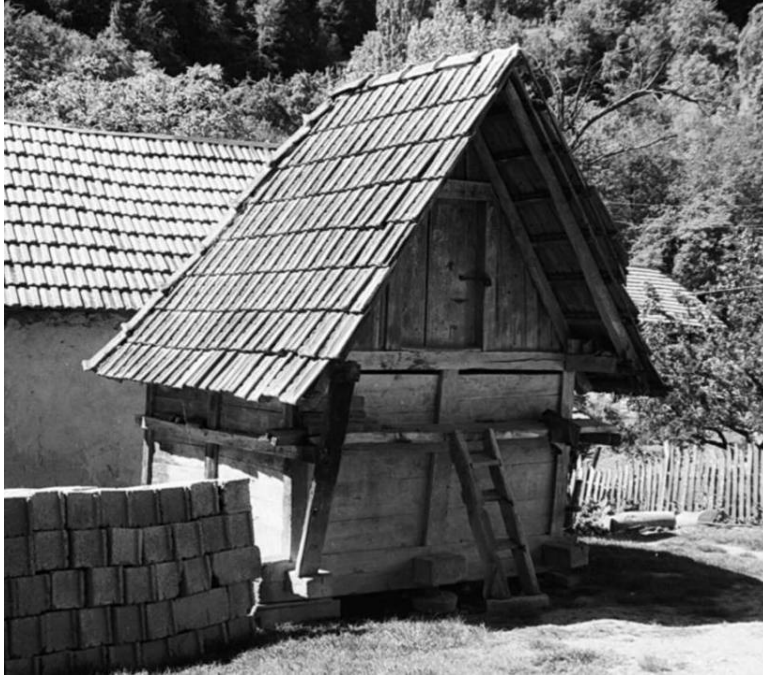
Figure 22. Granary with a wide front eave from the village of Godečevo (roof cover replaced)
