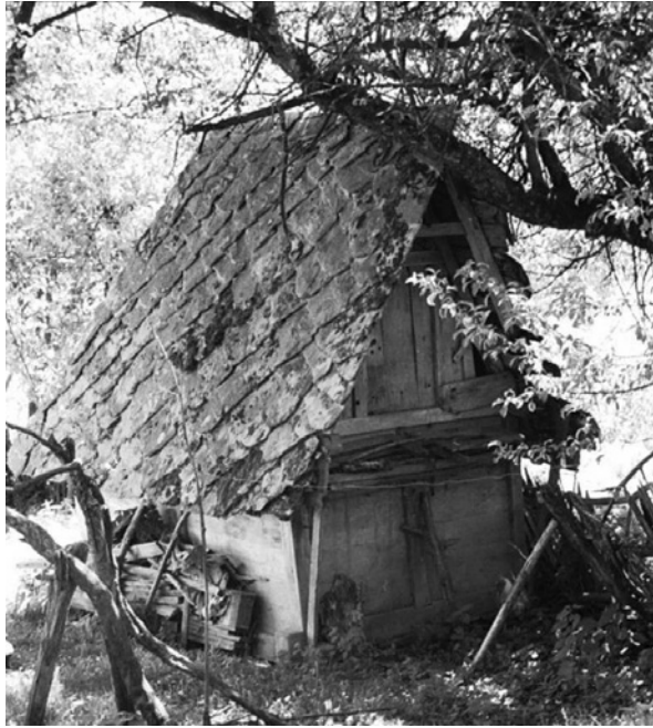
Figure 10. Granary covered by stone slabs from Godečevo
