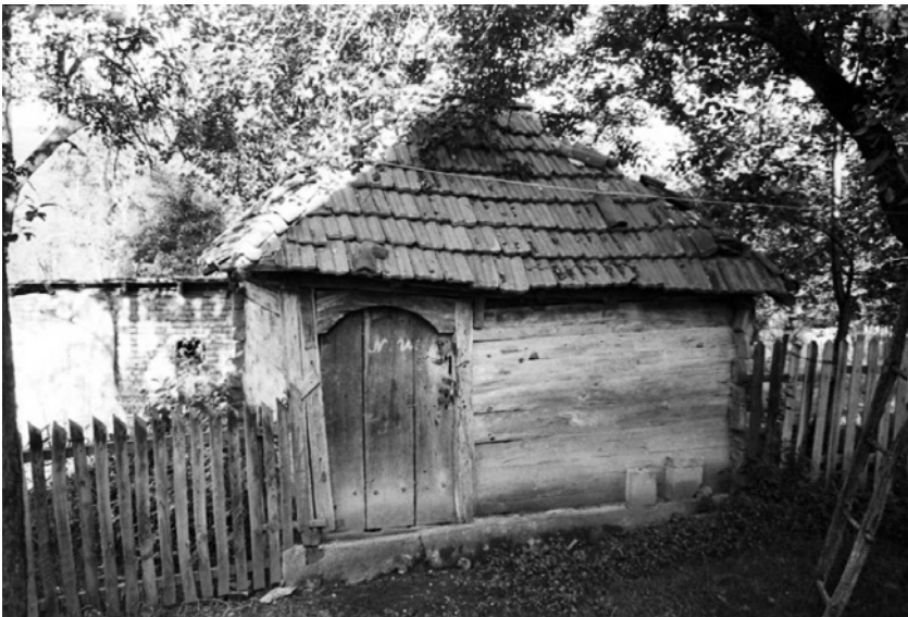
Figure 21. Vajat made wooden planks joined with tenon-and-mortise joint.
