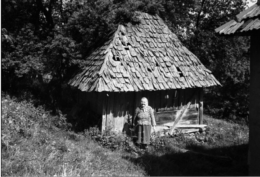
Figure 8. Vajat with a frame and (“na unizu”) tenon and mortise joints and wooden stips infill (“na šašovce”)
